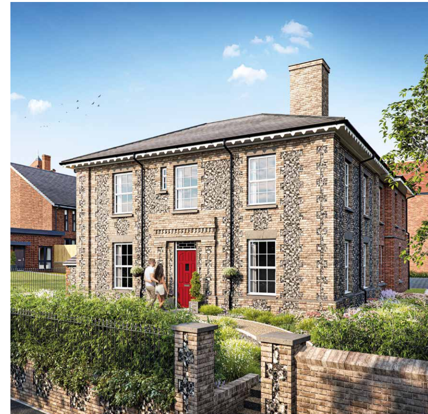
PLOTS 28-31 CROYDON BUILDING 1 & 2 BEDROOM APARTMENTS
